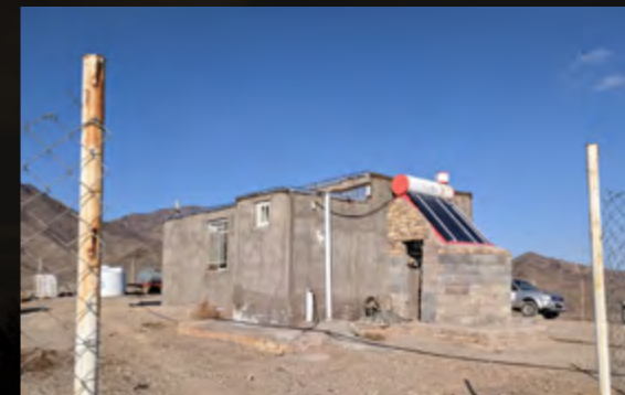
Jamil Station Under Construction
